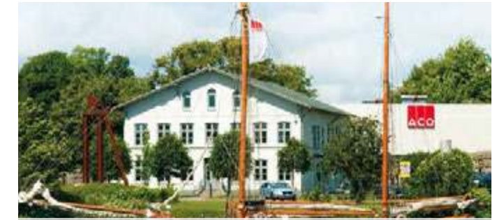
The historic building on the banks of the Eider river, the symbolic headquarters of the ACO Group
